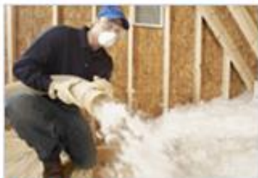
Blown In Insulation
